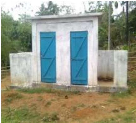
School Toilet of Babedpara
